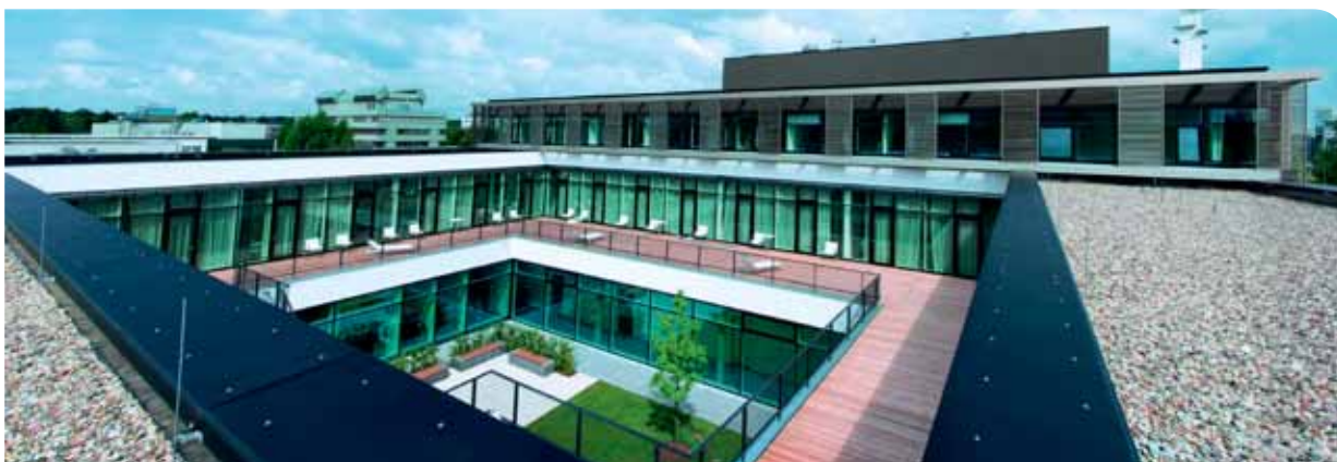
The new Clinical Research Center Hannover provides an interface between basic research and marketing authorization of new drugs and medical devices. © Fraunhofer/CRC Hannover
